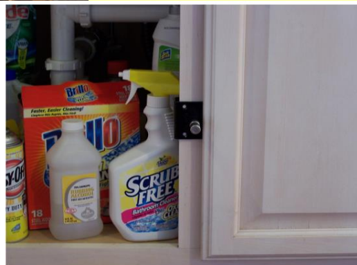
Slide bracket on and tighten thumb screws
